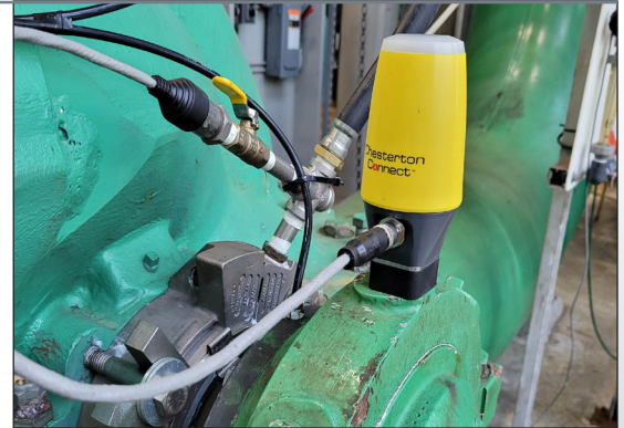
Chesterton Connect sensor connected to split case pump.
