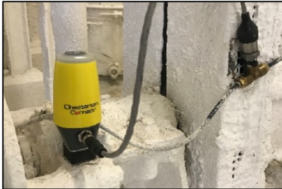
Chesterton Connect attached to slurry pump.
